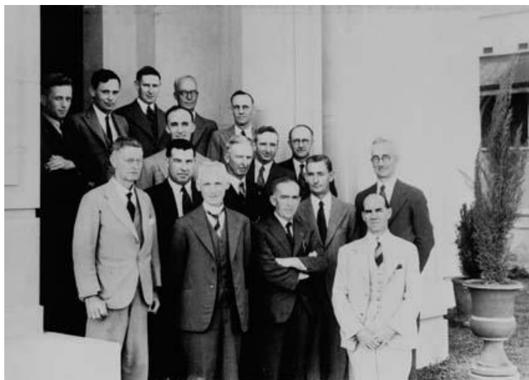
The opening of Rockhampton Automatic (Telephone) Exchange Building, 30 November 1940. Edward Lather is second on the left in the second row. He was divisional engineer in charge of country installations. At the left hand end of the second row is the Mayor of Rockhampton, Mr R W Evans
